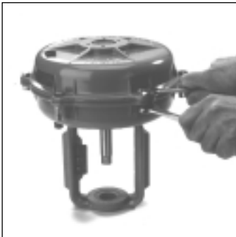
Fig 1 - Remove Housing Bolts
