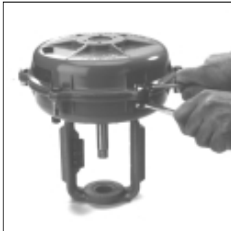
Fig 1 - Remove Housing Bolts
